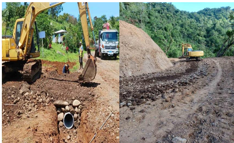
Figure 4.3.3.1 Roadworks in the Western Division
