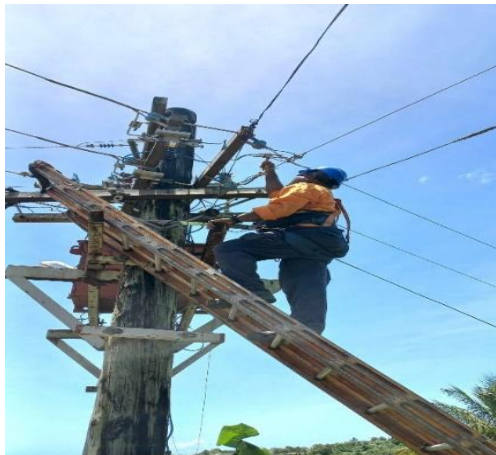
Figure 4.3.4.1 Nabouwalu Rural Government Station Powerlines Repair
