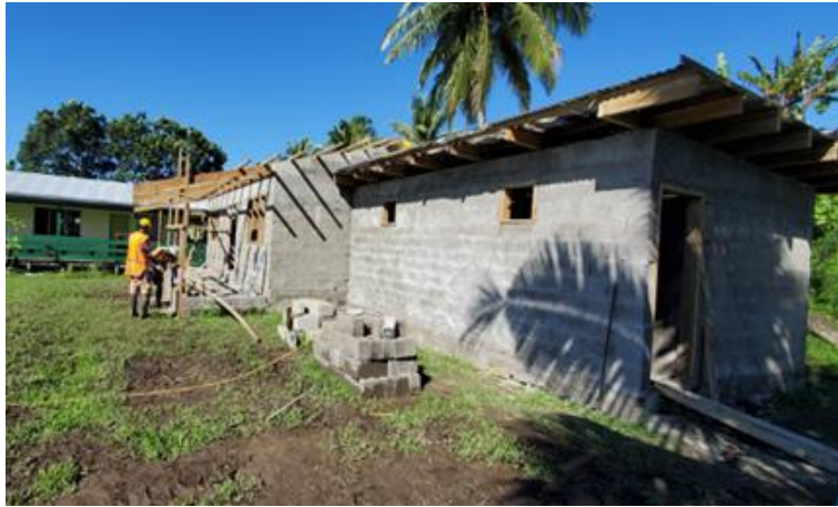
Figure 4.3.2.1 – Construction of ECE and Ablution block for Nasinu Gospel School
