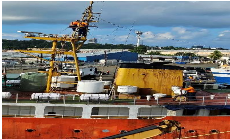
Figure 4.3.2.4 Repairs to GSS Boat
