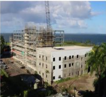
CARPENTERS- HILTON GARDEN Hotel development in Suva.
