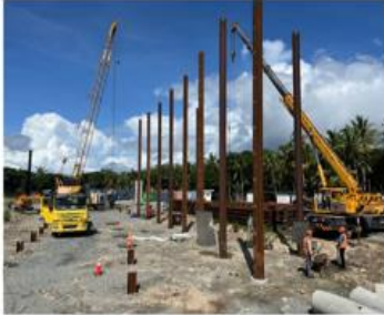
SOFITEL RESORT VATU TALEI New Extension-Vatu Talei 5-Star 190 Room.
