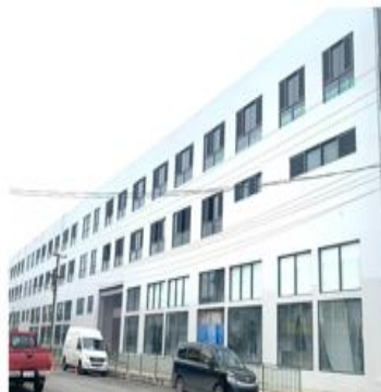
NAUSORI PLAZA Development of office space, restaurants, and shopping malls in Nausori.
