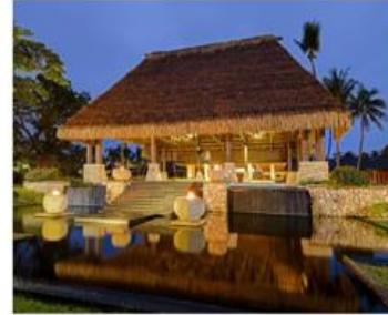
WESTIN FIJI Refurbishment of all 255 guest room, restaurants and public area.
