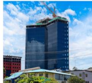
FHL TOWER 17-story commercial building in of Suva.
