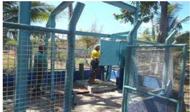
Figure 8: Inspection of WAF Wastewater Pump Station
