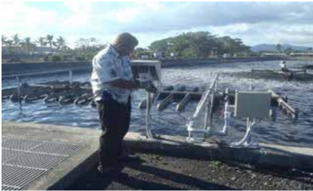
Figure 7: DWS Staff inspecting Navakai Wastewater Treatment System in Nadi
