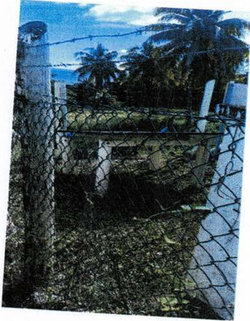
Mua VSAT Station
