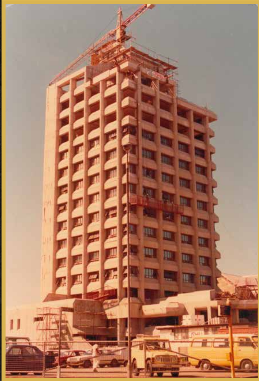
RBF Building under construction, opened on 27 July, 1984
